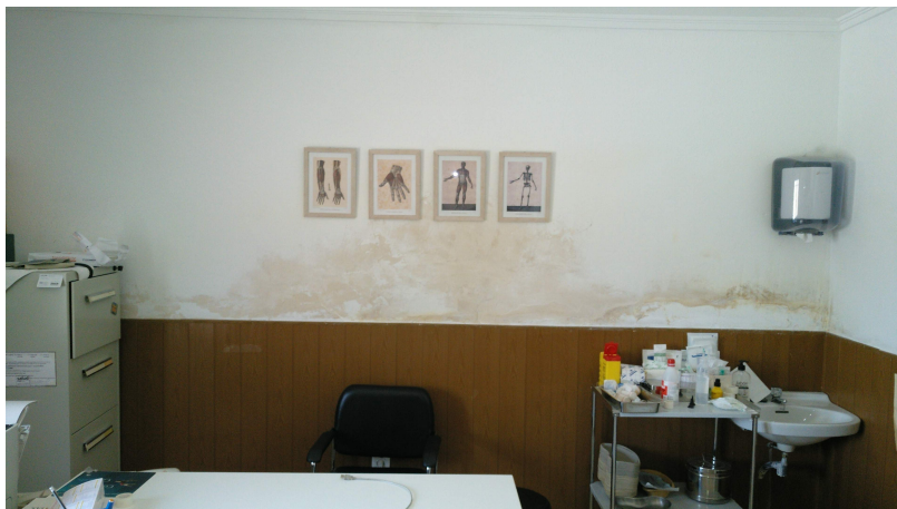
Vista general interior 1
